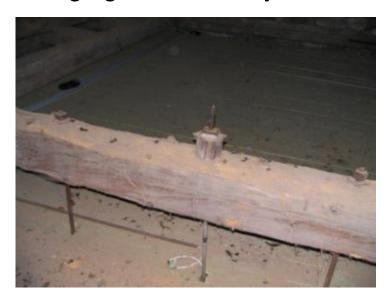
Suspension truss with medium threshold purlin
