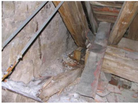
Because of vault, truss over the chancel is solved without tie beams vault has no signs of damage
