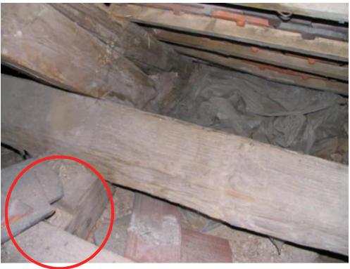
Some tie beams are in very poor condition and will require their total replacement
