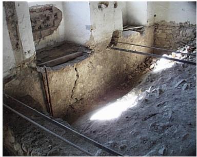
reinforcement of the building with prestressing steel draw rods
