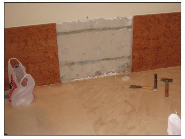
Depth core bore holes (Knapen channels)
